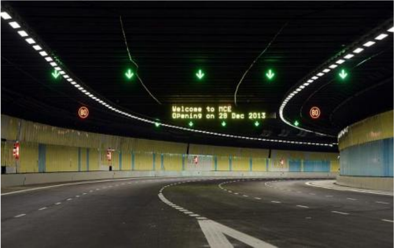
Figure 2.10: Intelligent transport systems with guidance from the interior: Marina Coastal Expressway Tunnel, Singapore
