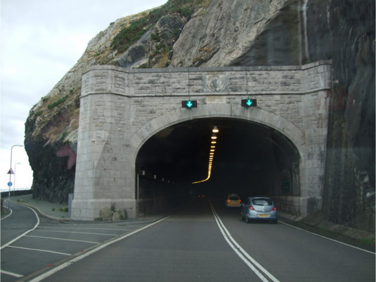
Figure 2.6: Example of lighting changes from A55 Pemaenbach Tunnel portal, Wales
