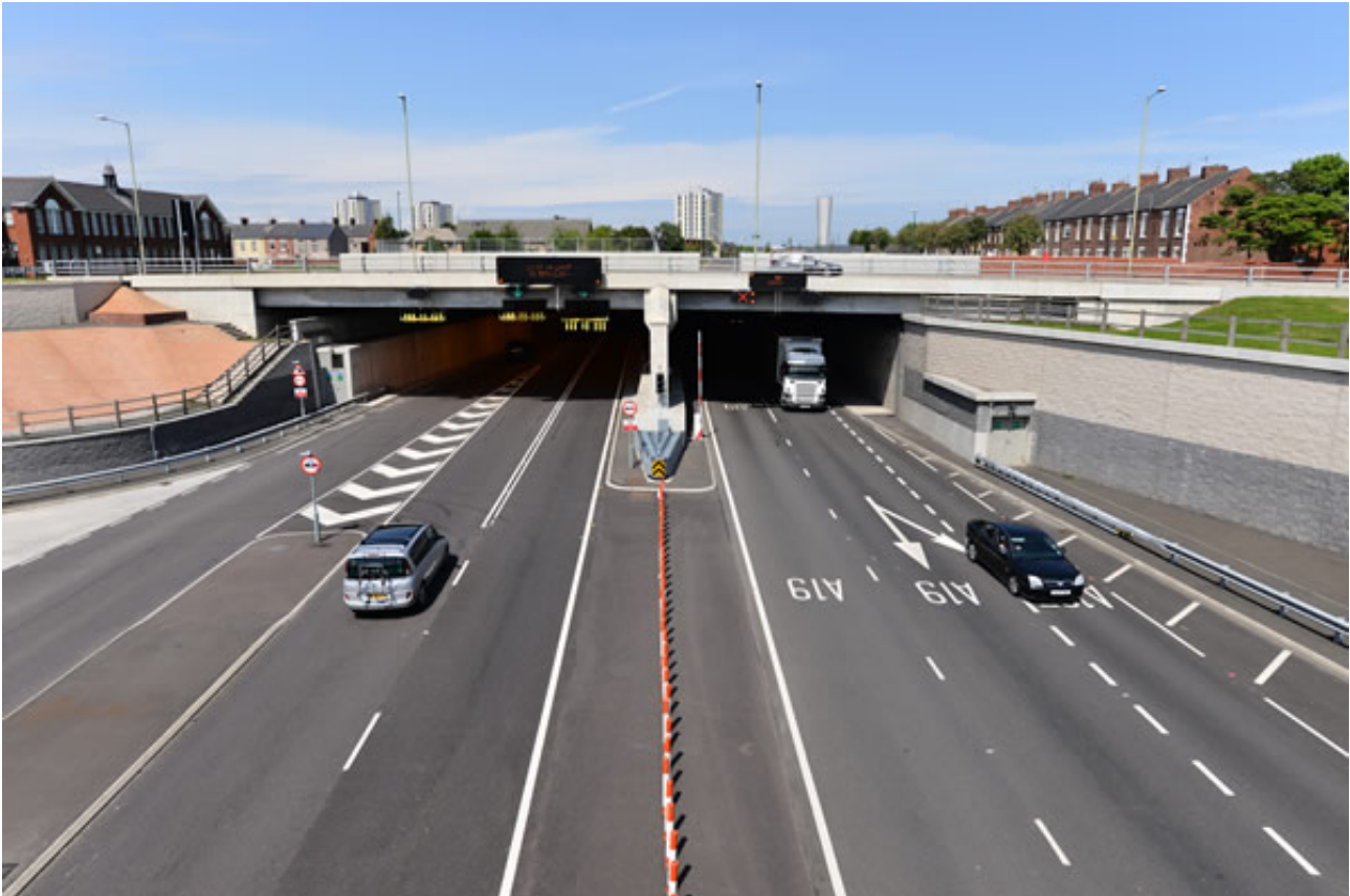
Figure 2.11: Tyne Tunnel portal – northbound: refurbished to ensure safety standards are met
