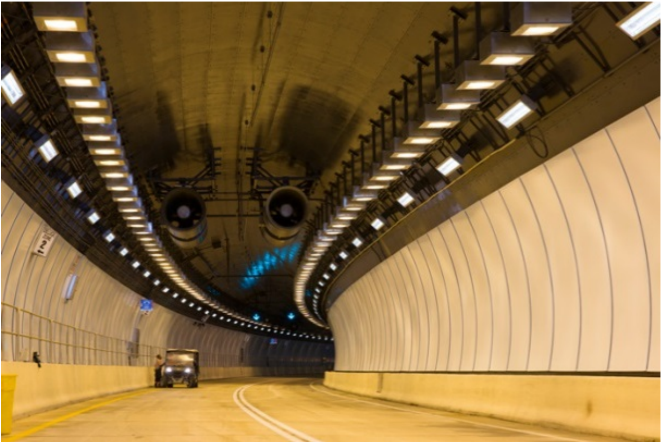
Figure 2.9: Proximity of lane to wall from the interior of Port Miami Tunnel (State Road 887), USA
