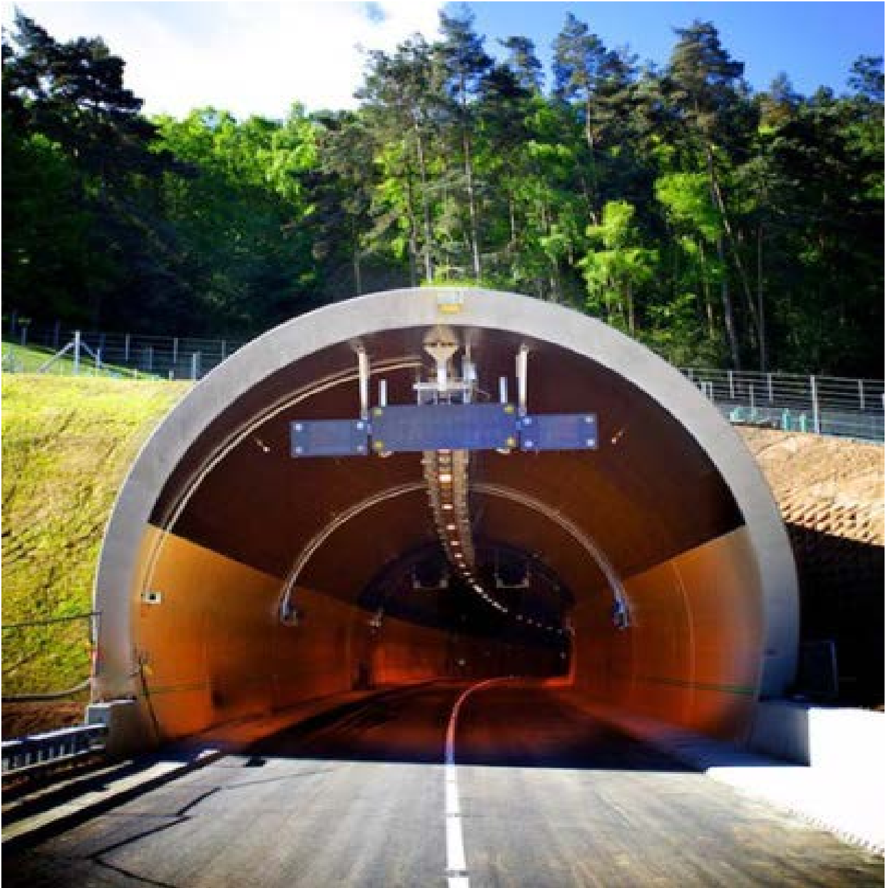
Figure 2.7: Tunnel entrance at A3 Hindhead Tunnel portal, England
