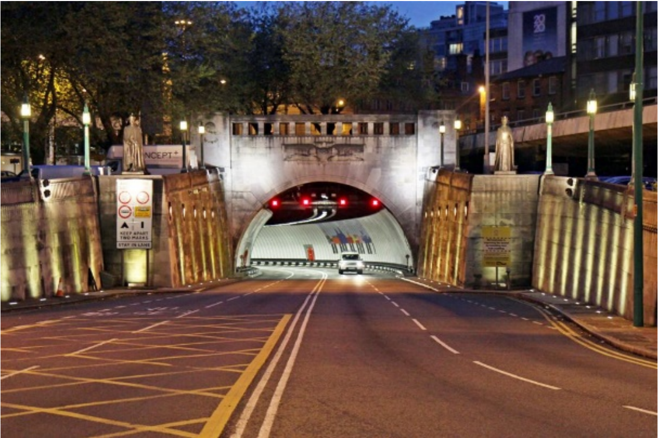
Figure 2.13: Mersey tunnel entrance with ITS implementation
