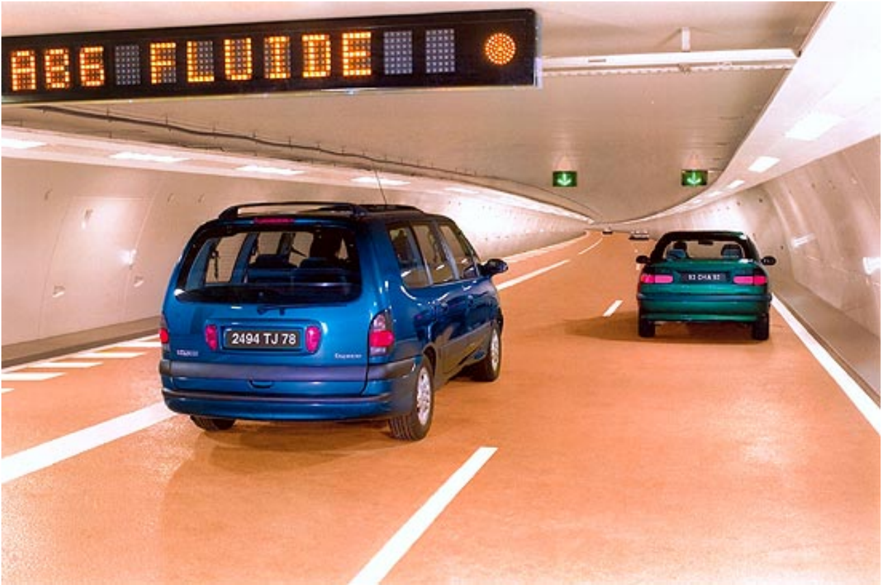
Figure 2.12: Interior of A86 West Tunnel, France showing ITS system in use
