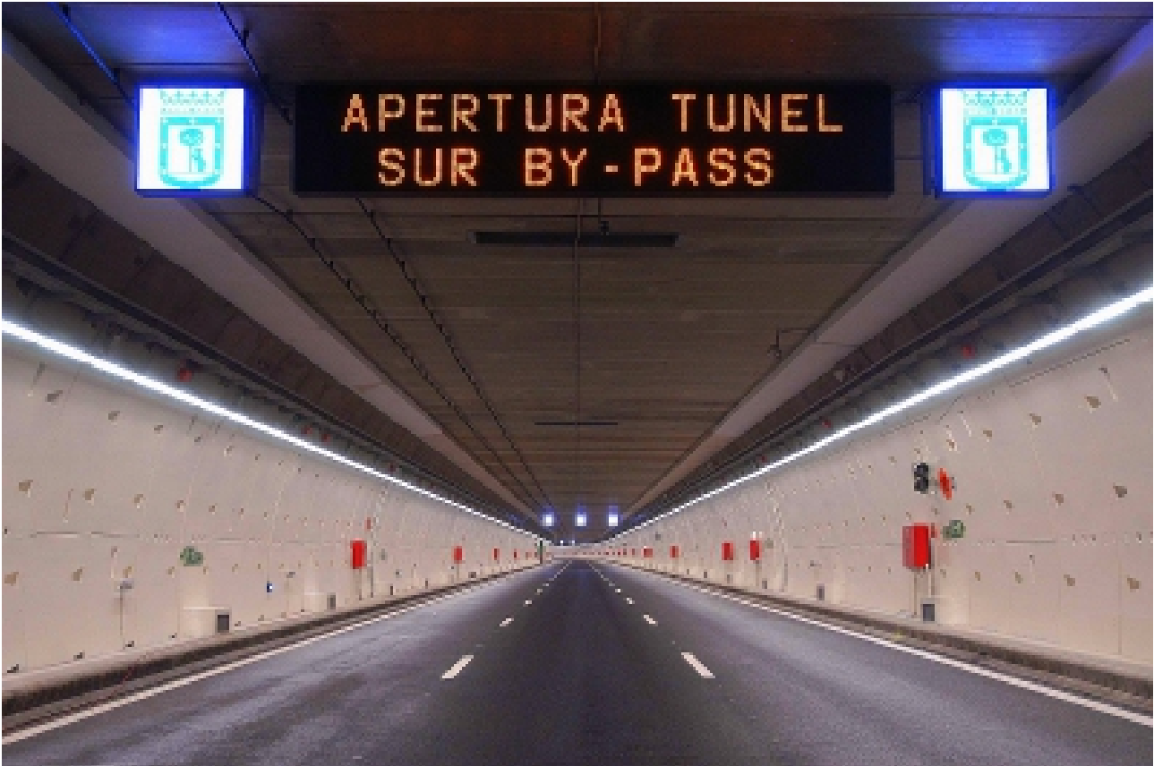
Figure 2.5: Lighter colour walls in the interior of Calle 30 Tunnel, Spain
