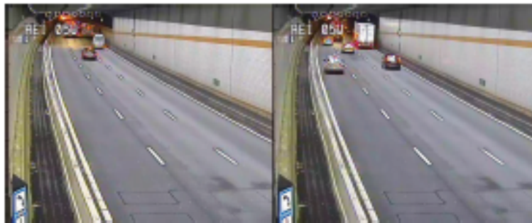
Figure 8 Tunnel portal at t = 0 sec (accident) and t = 15 sec when traffic stops
