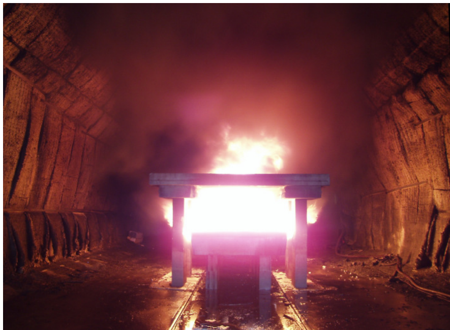
Figure 3: Fire Tests during UPTUN Program (Photo: Courtesy of FOGTEC, Germany)
